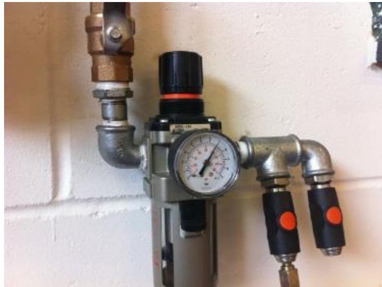
Figure 4-17 Air valve to adjust the pressure
