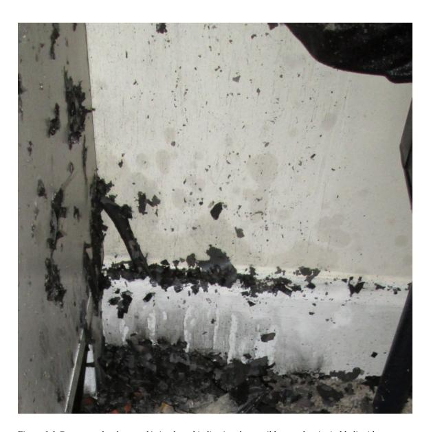
Figure 1.1 Greasy marks above a skirting board indicating the possible use of an ignitable liquid
