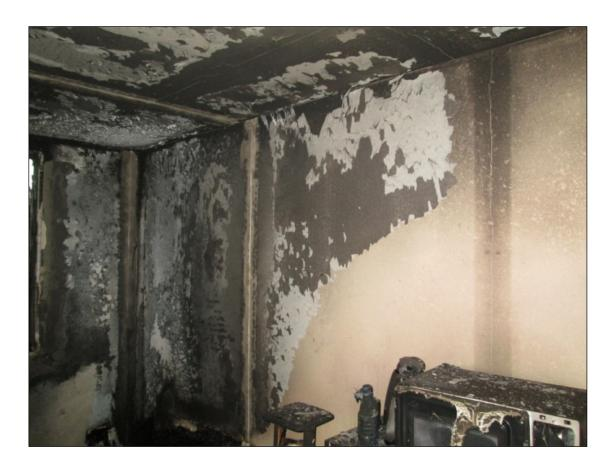
Figure 6.18 The area above the sofa with a 'V' shape on the plasterboard walls
