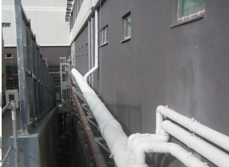
Rain water collection; the main pipeline hanged along the building walls as a ring line, collecting rainwater from each columns from roof to bottom.
