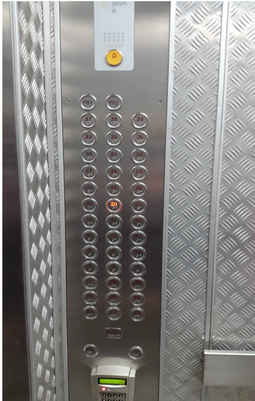
Figure 17: Missing Floors on Floor Indicator in Lift. (photograph permission of N Wilkinson)
